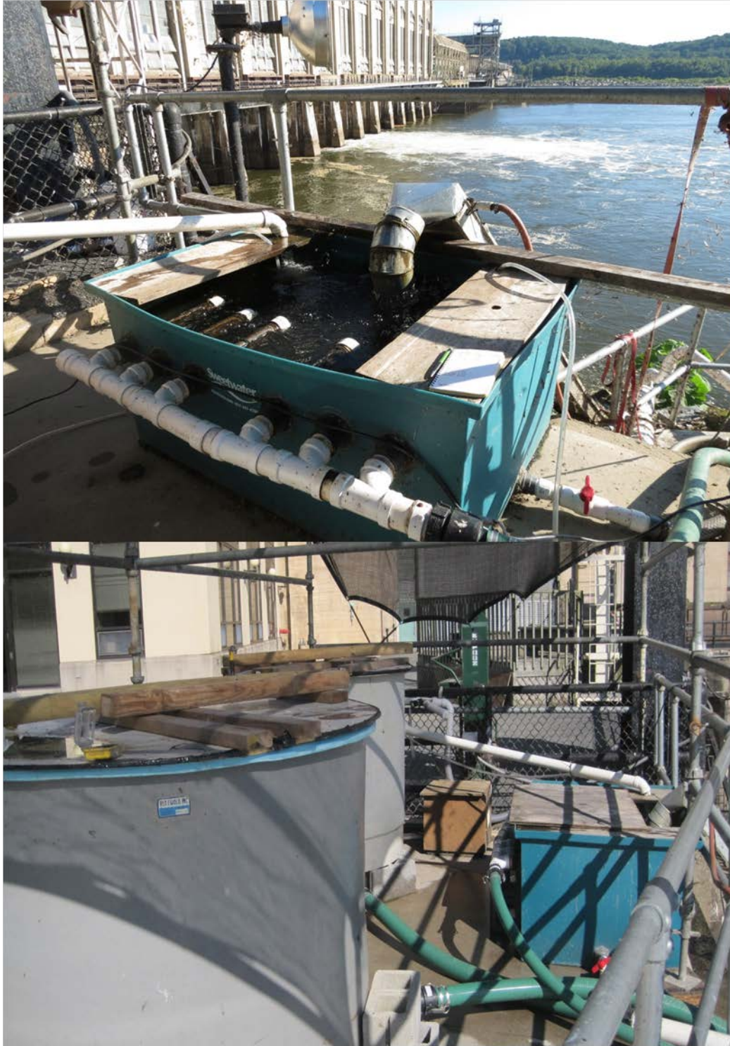
Figure 7. Collection tank and holding tanks located on the lower platform, at the top of the elver ladder, Conowingo Dam, Maryland. Photo credit to USFWS/MFRO/JMalavasi.
